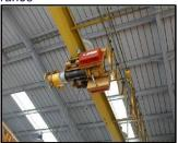
**Trolley Mounted Overhead Hoist**
